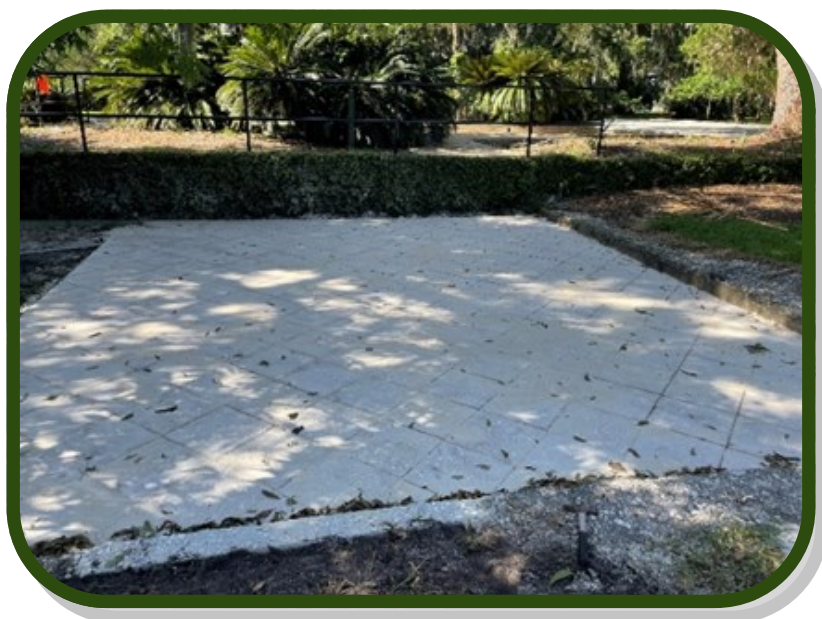
Work being done on Chichota Ruins
